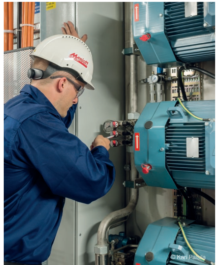
Part of the annual maintenance is to check pressure switch settings.
