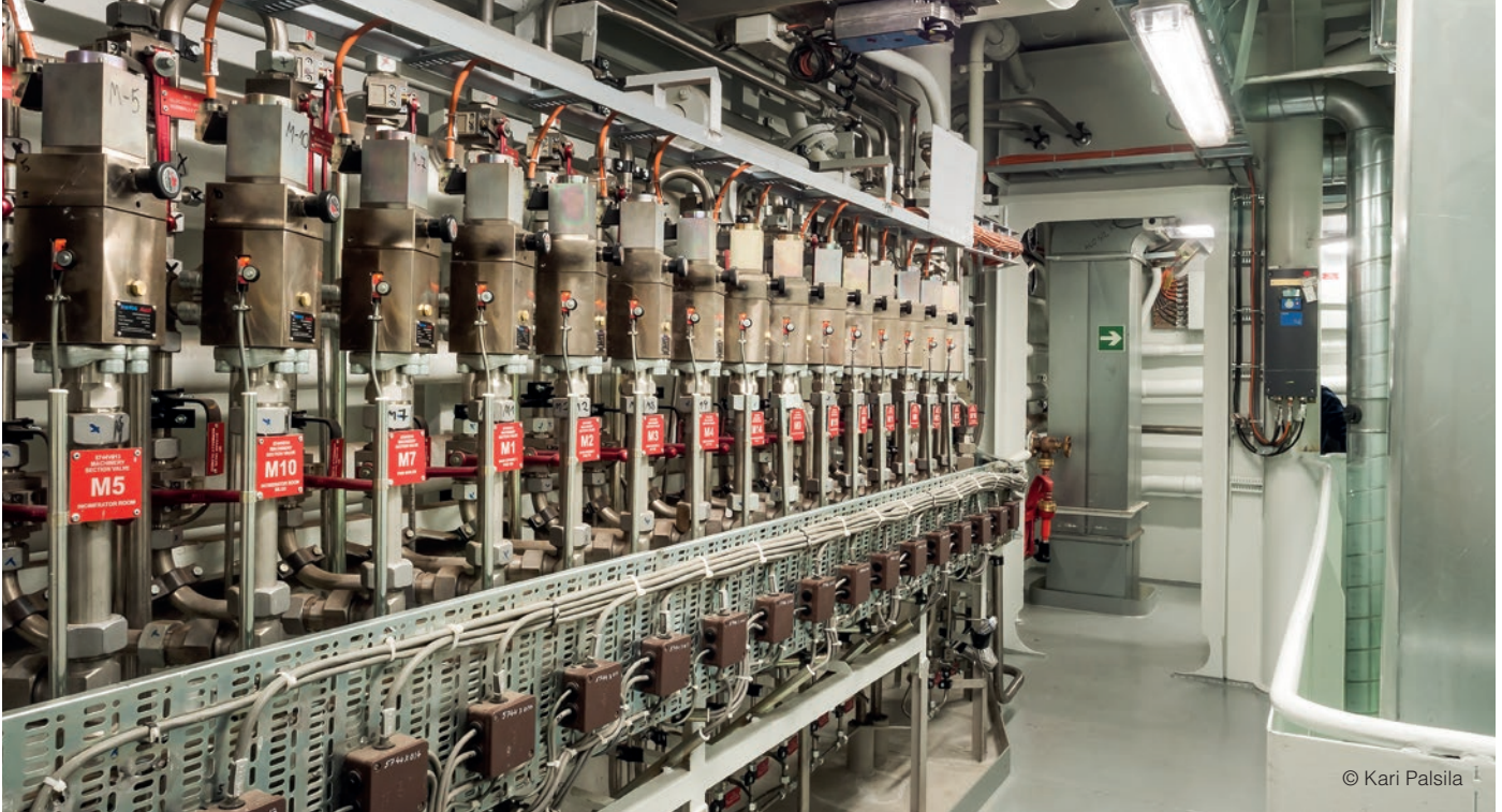
Good example of multiple machinery installation. All machinery valves are easily accessible for operation and maintenance.
