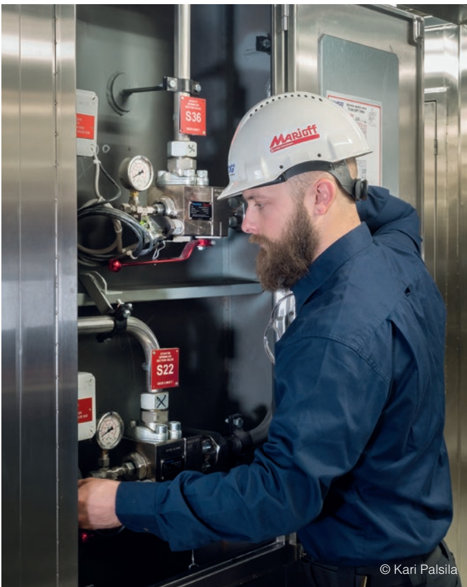
Valve signal testing is part of the Mariott's annual service. Installation inside the cabinet protects the valves and offers clean-cut interior.
